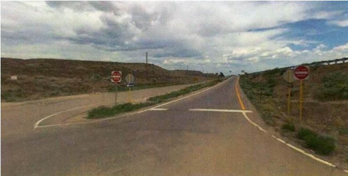
Figure 8. End of exit ramp 122, possible wrong-way driver entry point for the Fountain, Colorado, collision.
